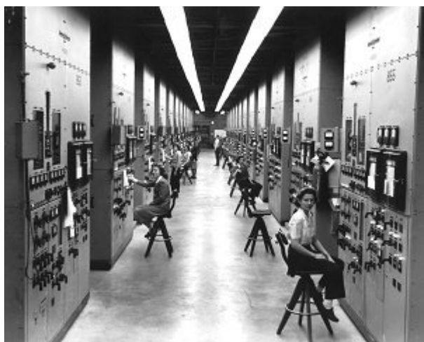
Young female cubicle operators monitor the activity of the calutrons, the heart of the uranium electromagnetic separation process at the Y-12 plant. Courtesy of Ed Westcott
